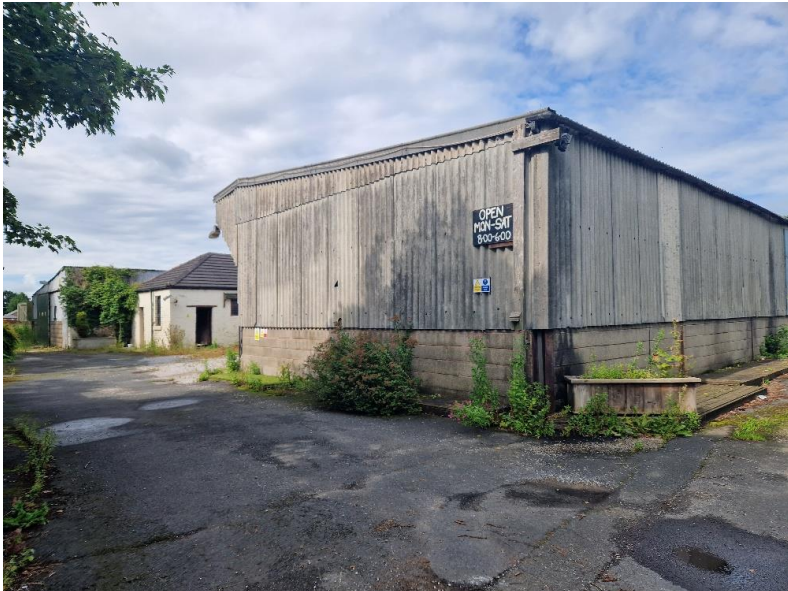
Photos of the Existing Site
